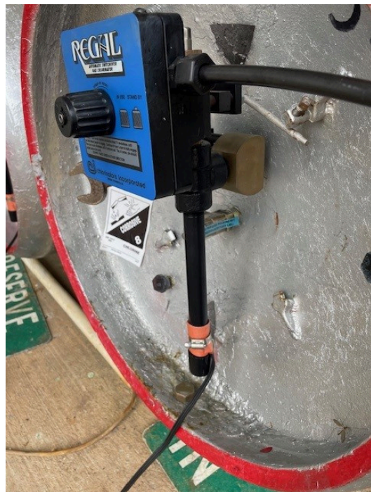
Ton Container Adaptor Assembly
